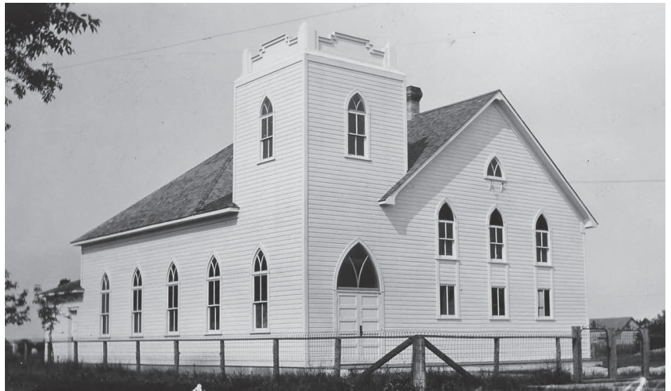
The Bruderthaler Mennonite church in Steinbach. Brandt produced the architectural drawings for the building. The Bruderthaler church was a forerunner to the Evangelical Mennonite Brethren Church (MAID MHC 720-96).
