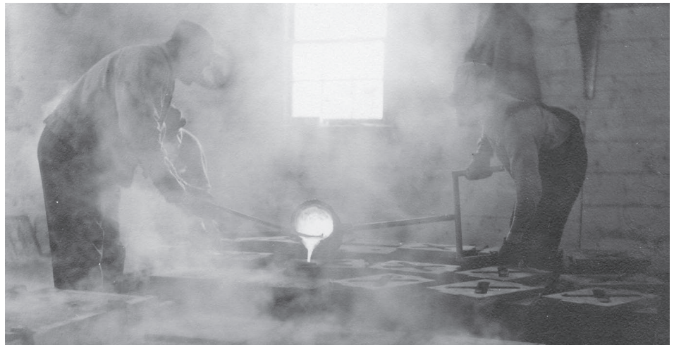
Workers pour molten metal into sand castings in the Brandt foundry (MAID MHC 720-05).
