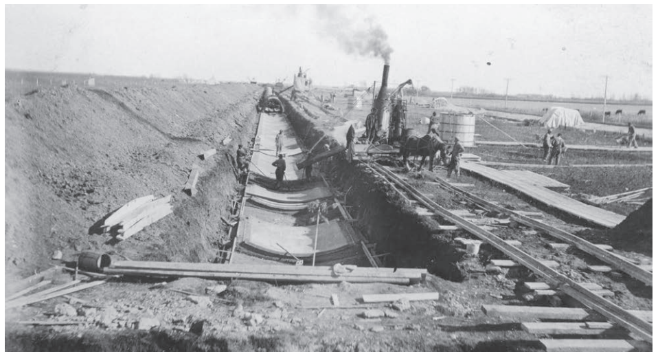
Aqueduct under construction, showing temporary railway tracks and horse-powered machinery (MAID MHC 720-29).
